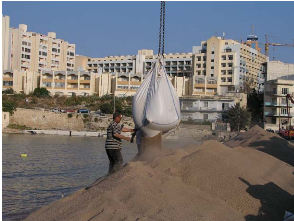
Figure 2: Beach replenishment work at St George's Bay (2004)
