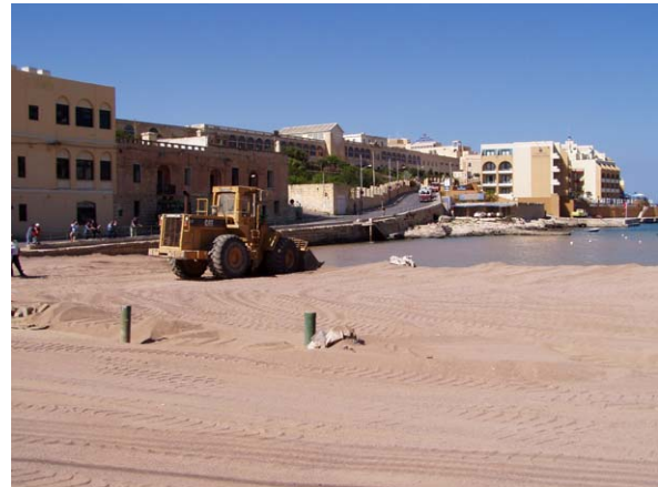
Figure 2: Beach replenishment work at St George's Bay (2004)
